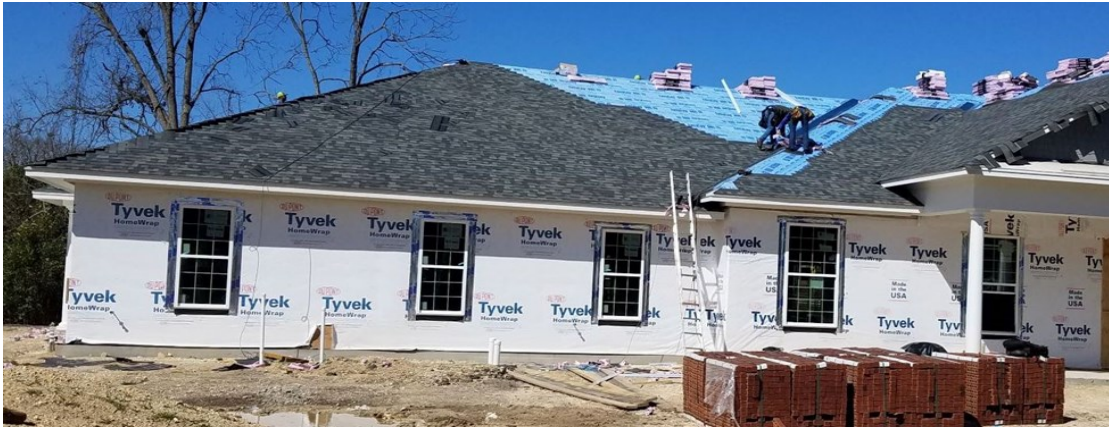
Amy's House under construction
