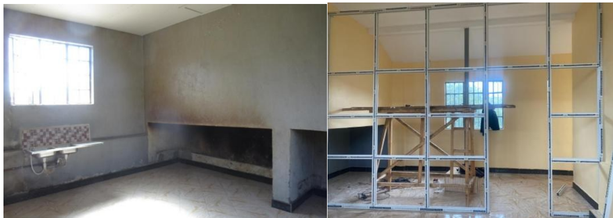
Works on the Dental Clinic in the Kibao Medical Centre
